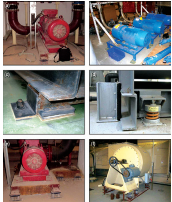
Figure 1. Six examples of poor vibration isolation system design from a conceptual perspective. The concepts in a-d undermine the isolator by shorting. The concepts in e and f potentially introduce unintended dynamics via weight distribution.
